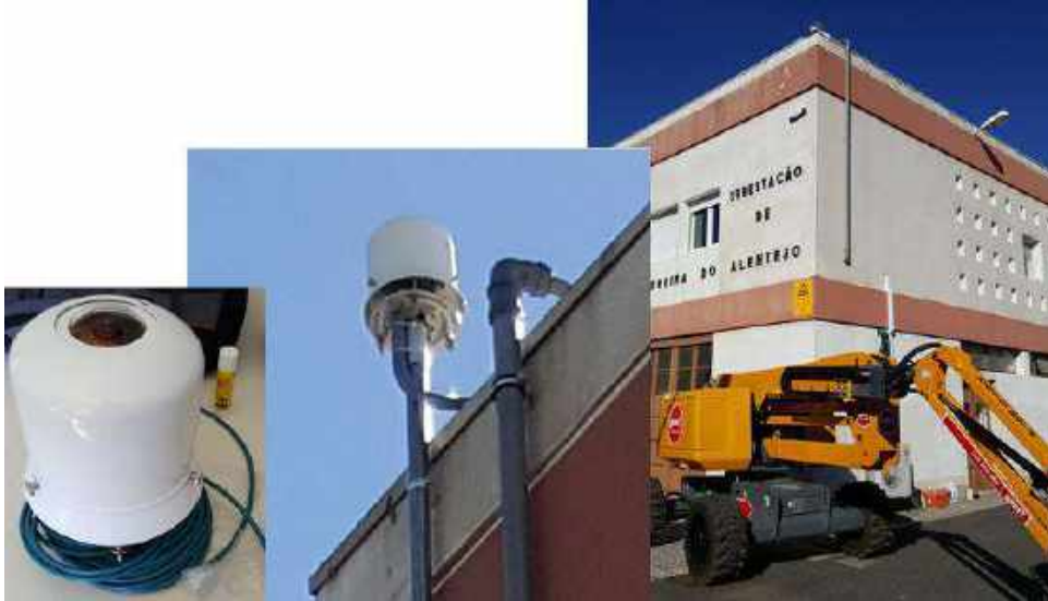
Figure 3 – Sky Camera in REN Substation
